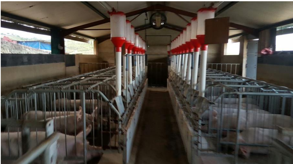
50-sow unit with automated water and feeds
