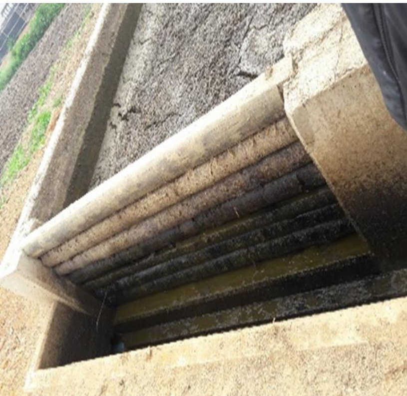
Wailing wall separating manure solids from liquid before solids are spread with Muck Spreader and liquid pumped through centre pivot into the pastures (waste recycling).
